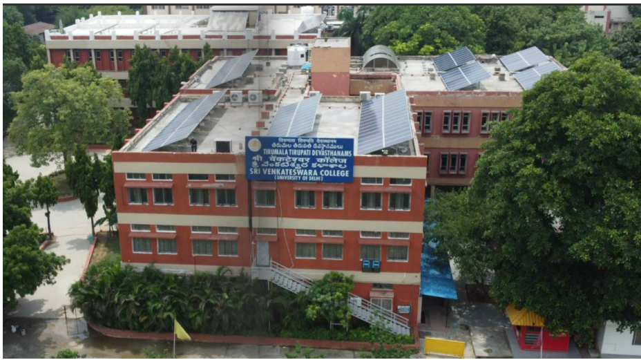
Drone View of Solar panels installed at Sri Venkatewara College
