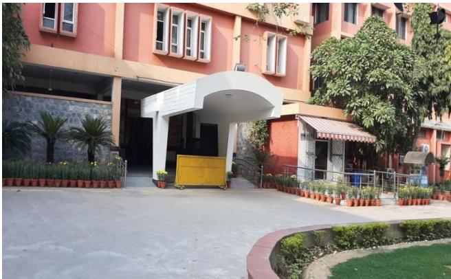
Ramp at entry to college building
