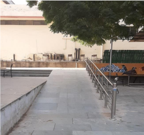
Ramp at the Cafeteria
