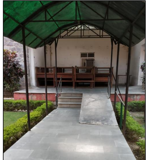
Ramp at entry to a classroom
