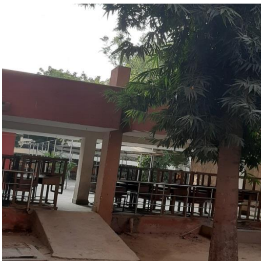
Ramp at entry to Photocopy facility
